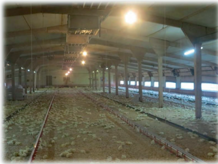
Figure 47 Shows inside House B
