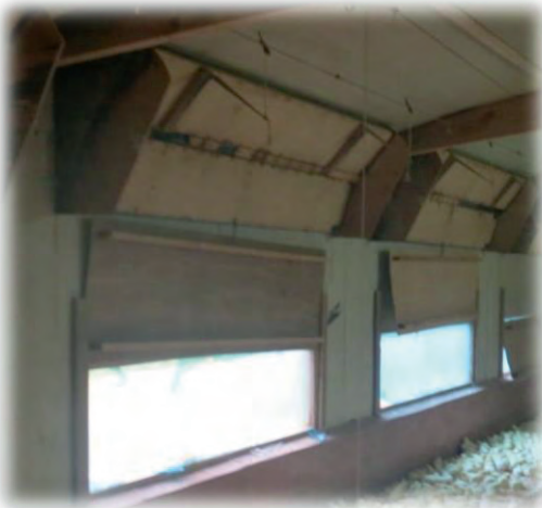
Figure 20 shows a very old-style manual inlet
