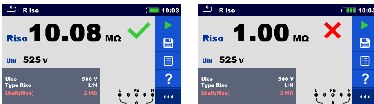
Figure 7.9: Examples of Insulation resistance measurement result
