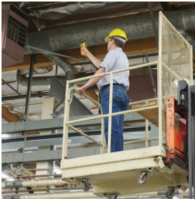
Identifying the temperature of ceiling-mount equipment.
