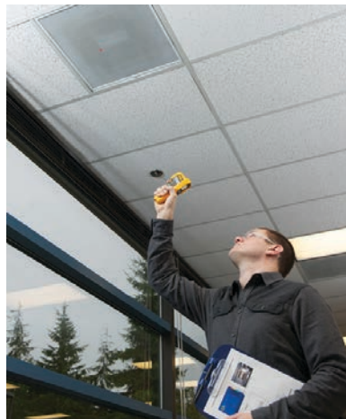
Checking the discharge temperature at air distribution ducts.
