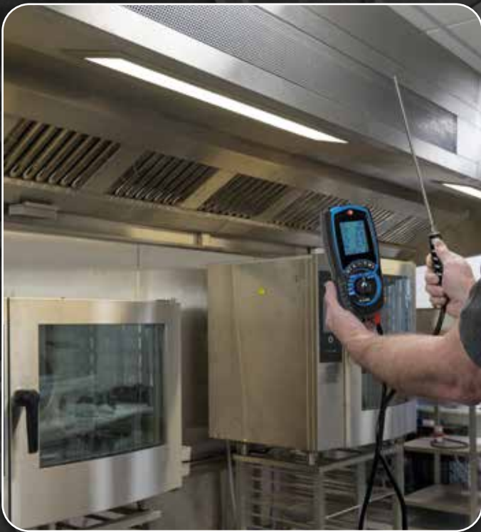
Monitoring Indoor Air Quality
