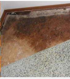
Leak Under The Floor
